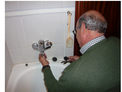
Image courtesy of SWITCH. © SWITCH Project
