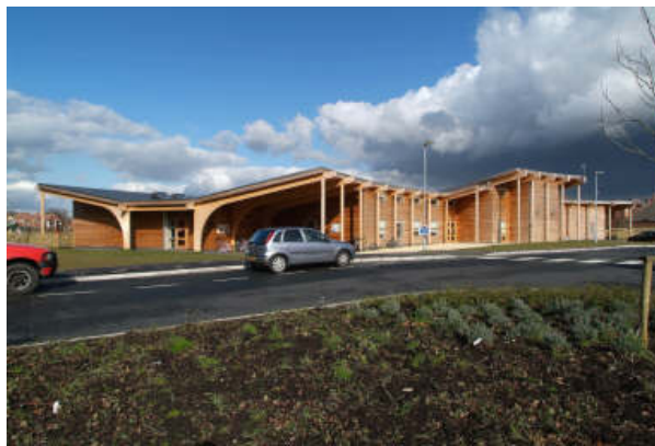
Figure 2.11 Kingsmead School, Cheshire, England
