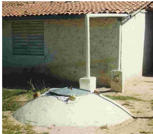
Figure 2.6 Water storage tank, Petrolina, Brazil
